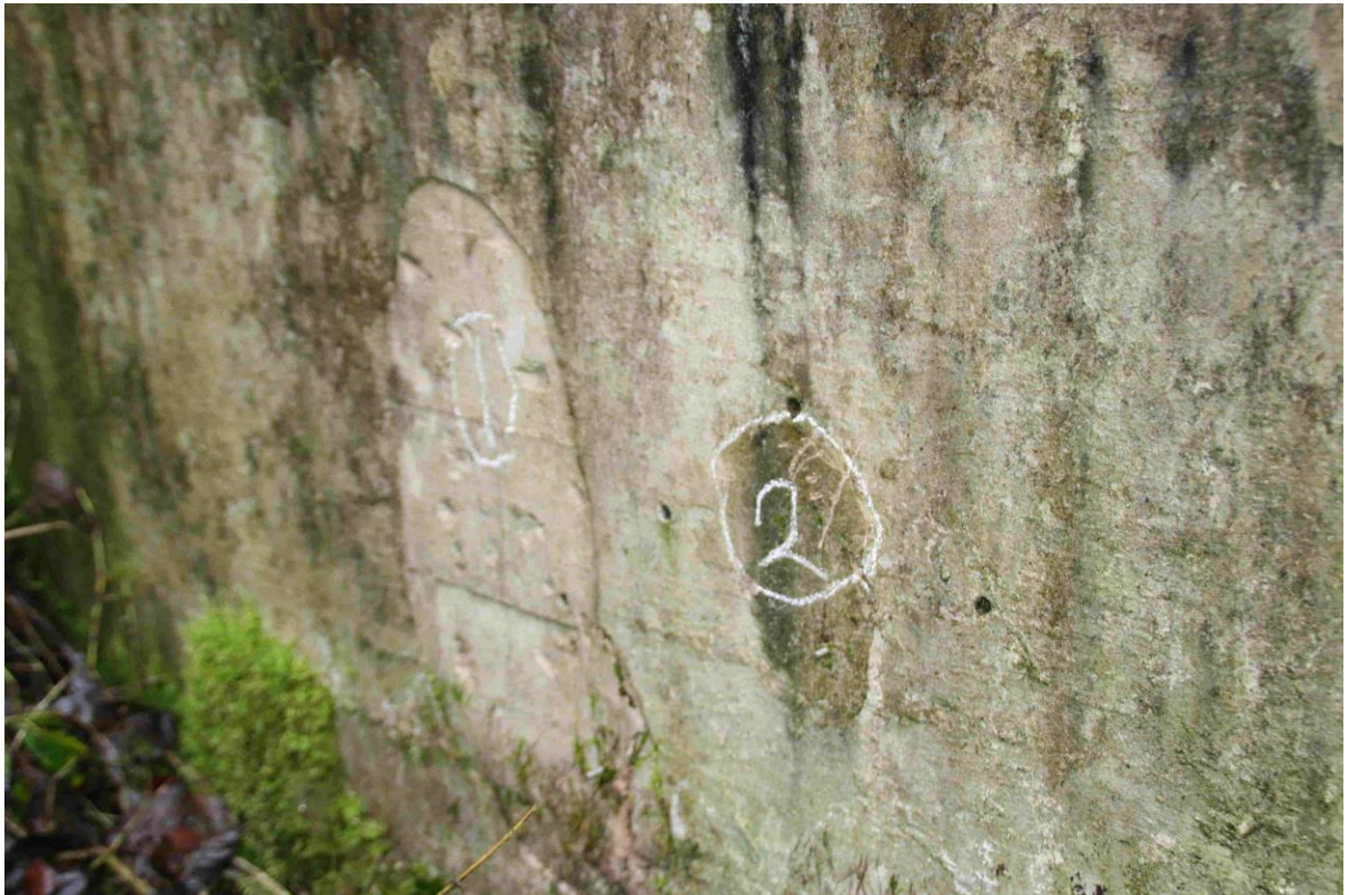
Figure 7 View of the small patch repairs (1 and 2) on the outer wall at 1 st floor level. Patch 1 was made using a proprietary repair mortar and patch 2 was made using a like-for-like concrete repair.
