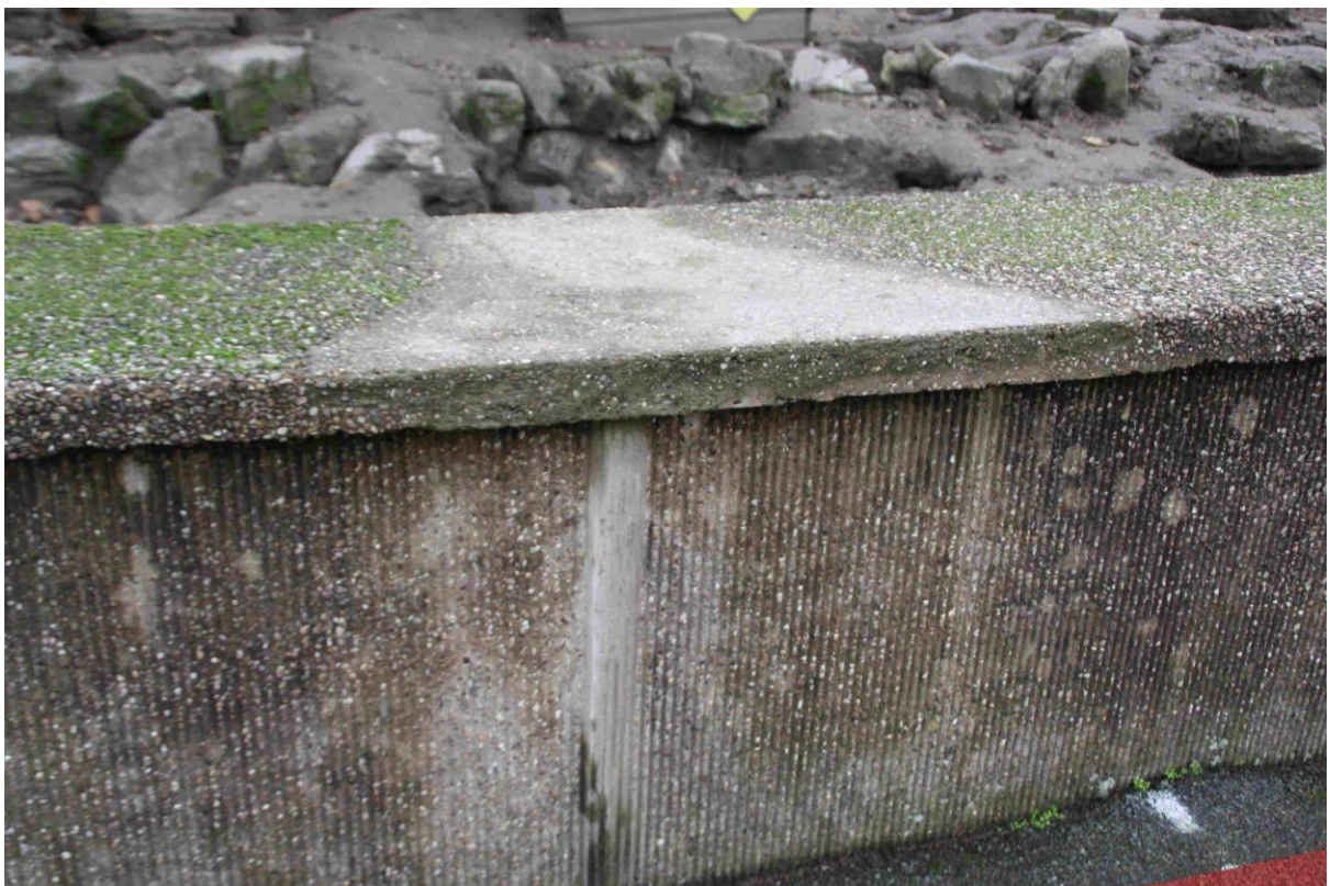
Figure 11 The repairs to both the top section and vertical fluted section have now weathered and have blending in with the parent concrete.
