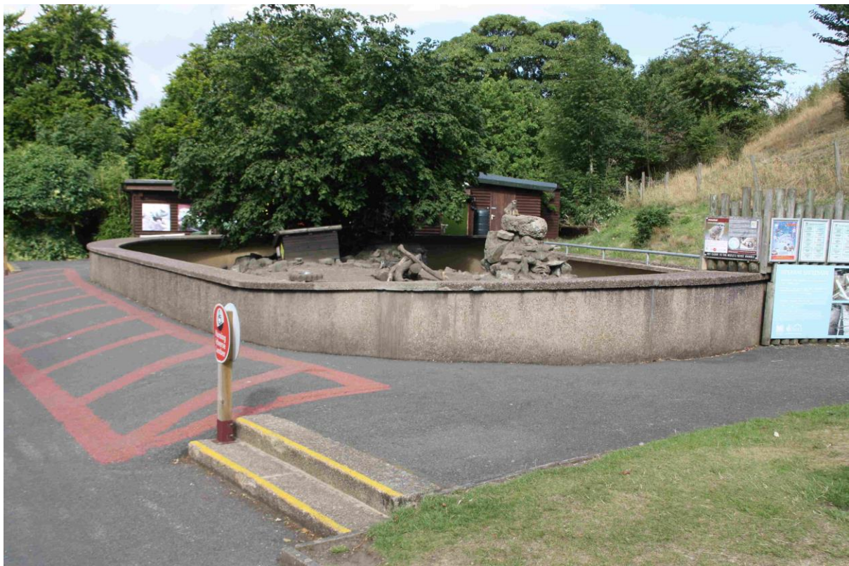
Figure 10 View of the repaired Meerkat Enclosure taken 7 years after completion.
