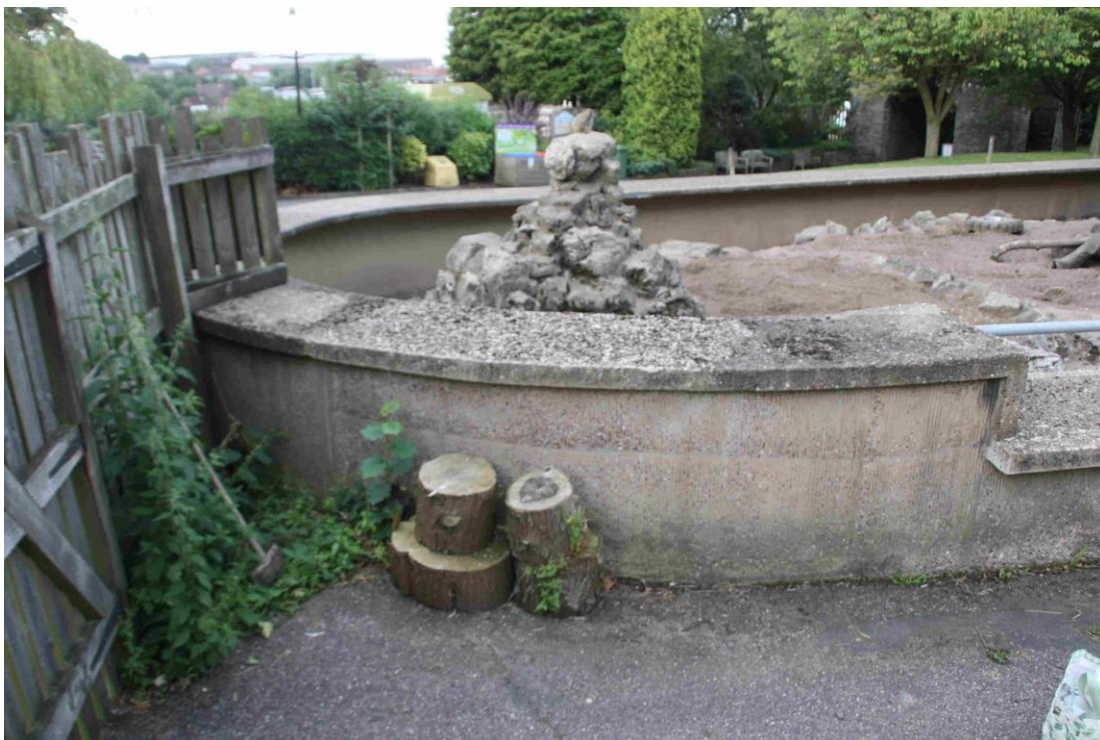
Figure 14 View of the repaired top of the wall showing it fully blending in after 7 years exposure.
