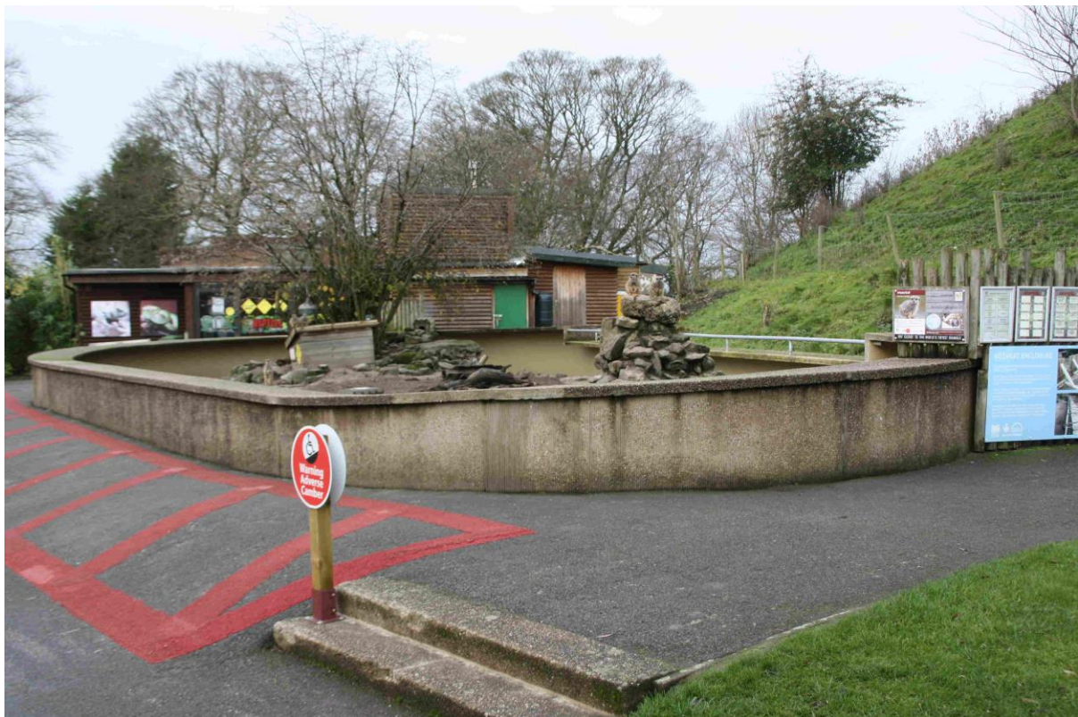
Figure 10 View of the repaired Meerkat Enclosure taken 5 years after completion.
