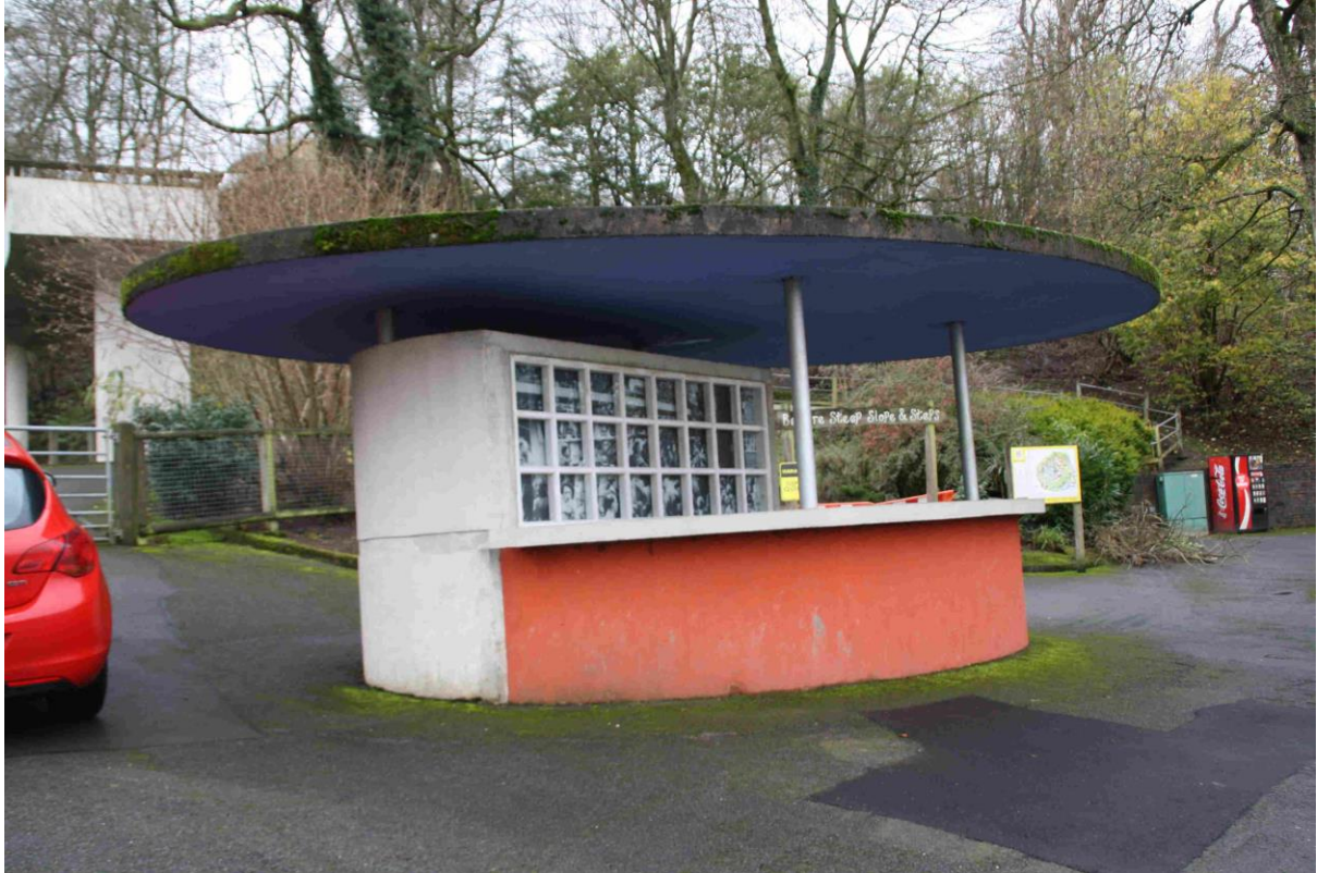
Figure 1 View of the repaired Kiosk after 7 years exposure.
