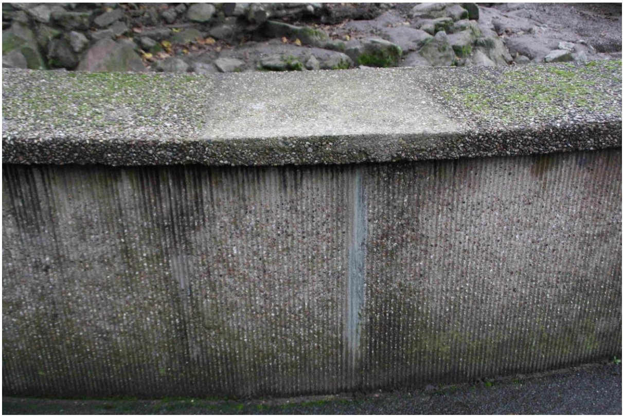
Figure 11 The repairs to both the top section and vertical fluted section are now blending in with the parent concrete.
