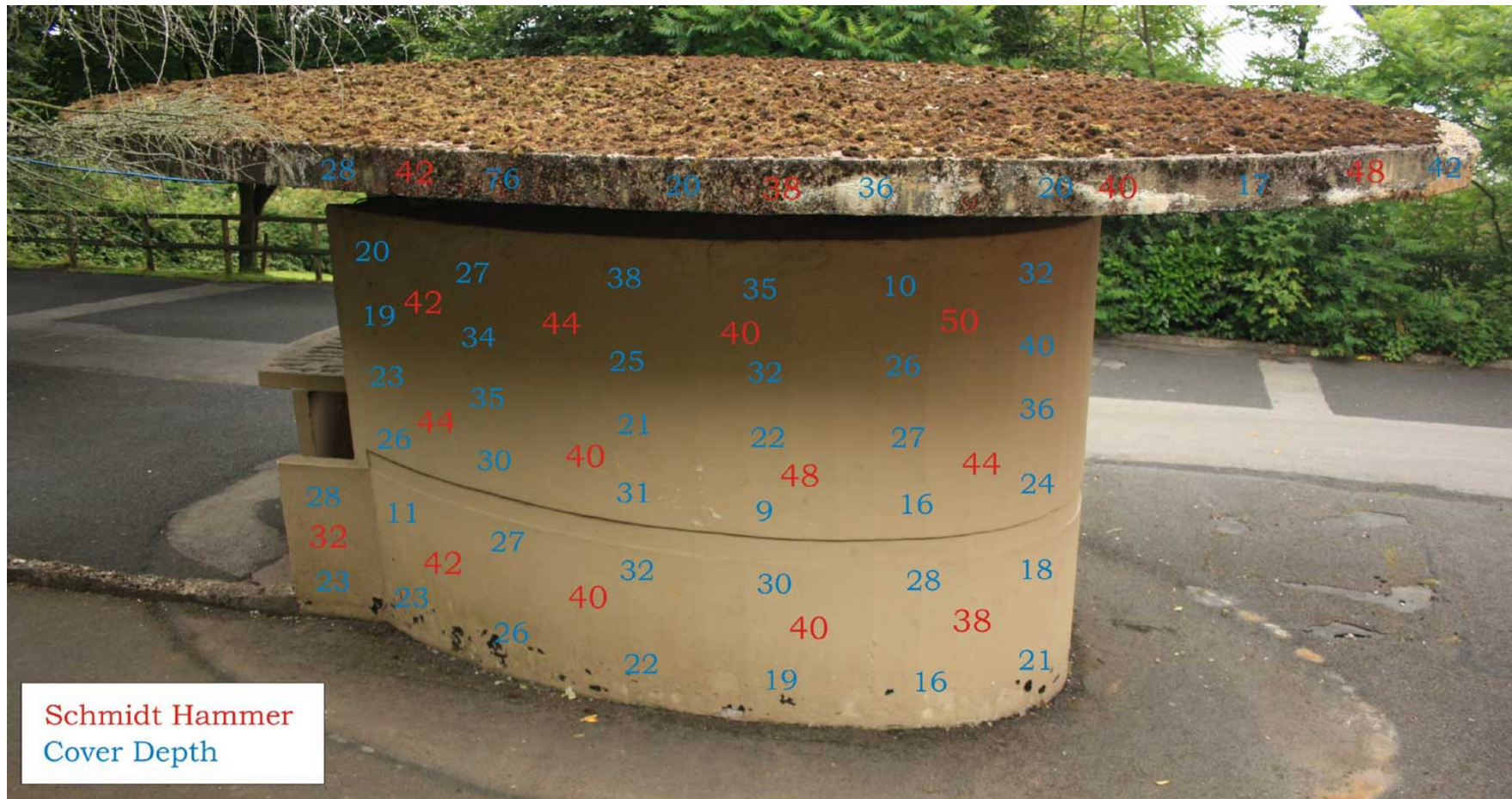
Figure A-12: Rear of Kiosk
