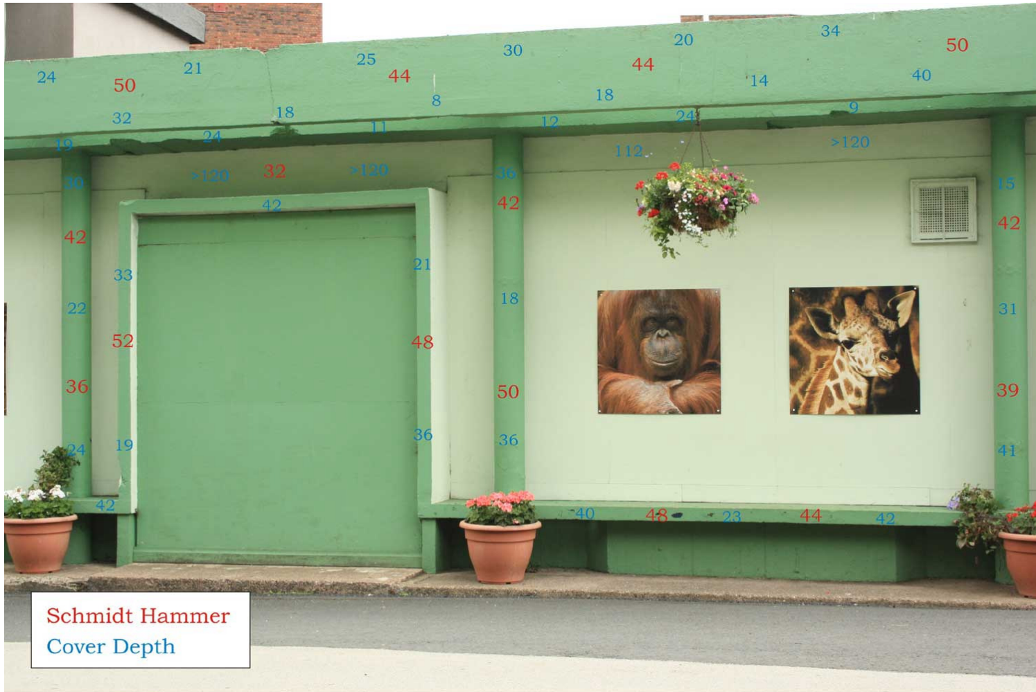
Figure A-19: Right side of the night club building (Area B)
