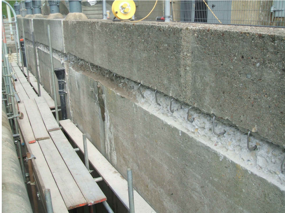
Figure C-3 Stainless steel cramps being inserted in the breakouts to bond the two concrete layers together and assist the mechanical bond of the repair.
