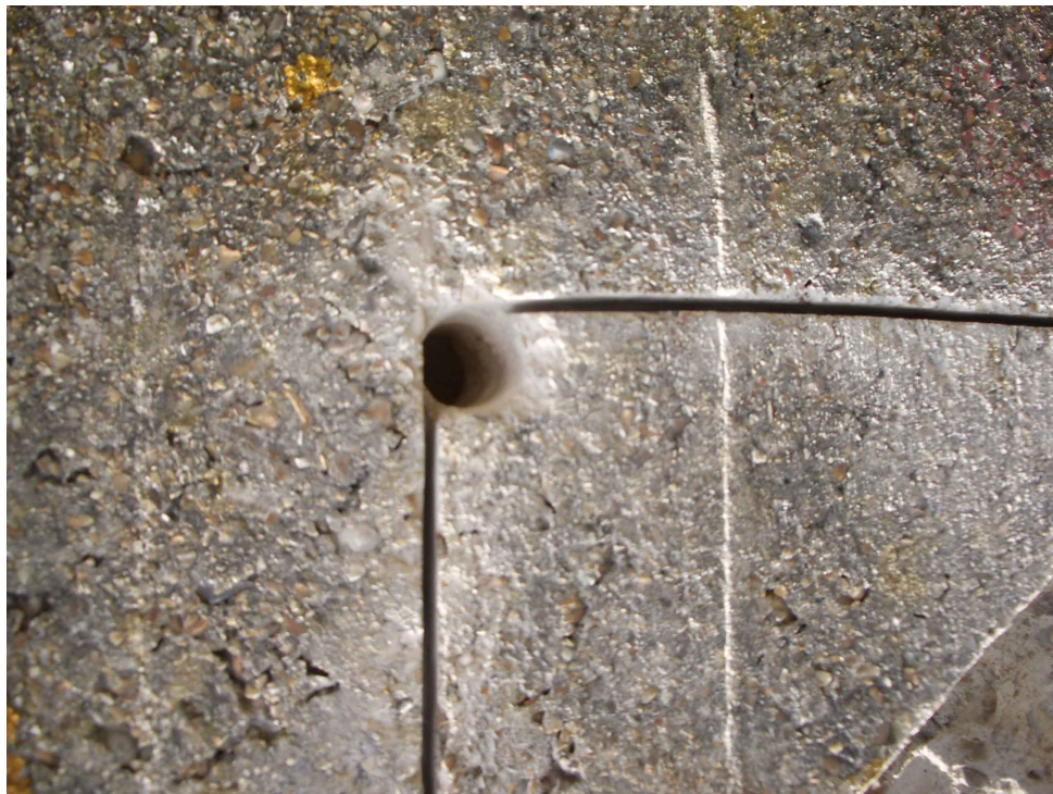
Figure C-2 Core drilling of the corners of the breakouts and dovetail cuts between to achieve additional mechanical fixing of the repairs.
