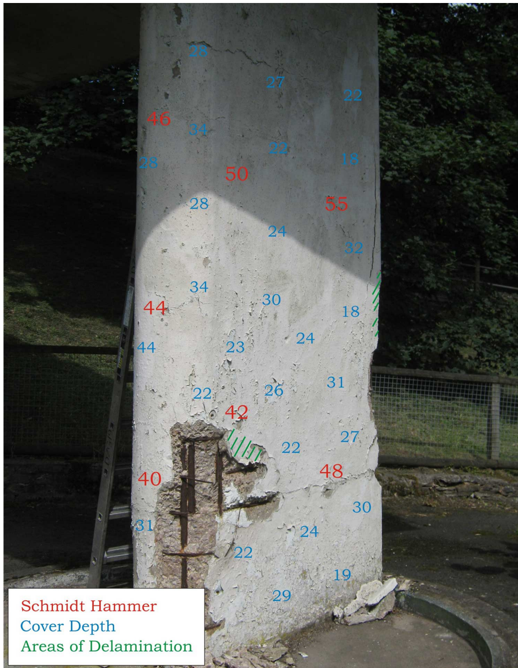
Figure A-9: End Column Wall (Area H)
