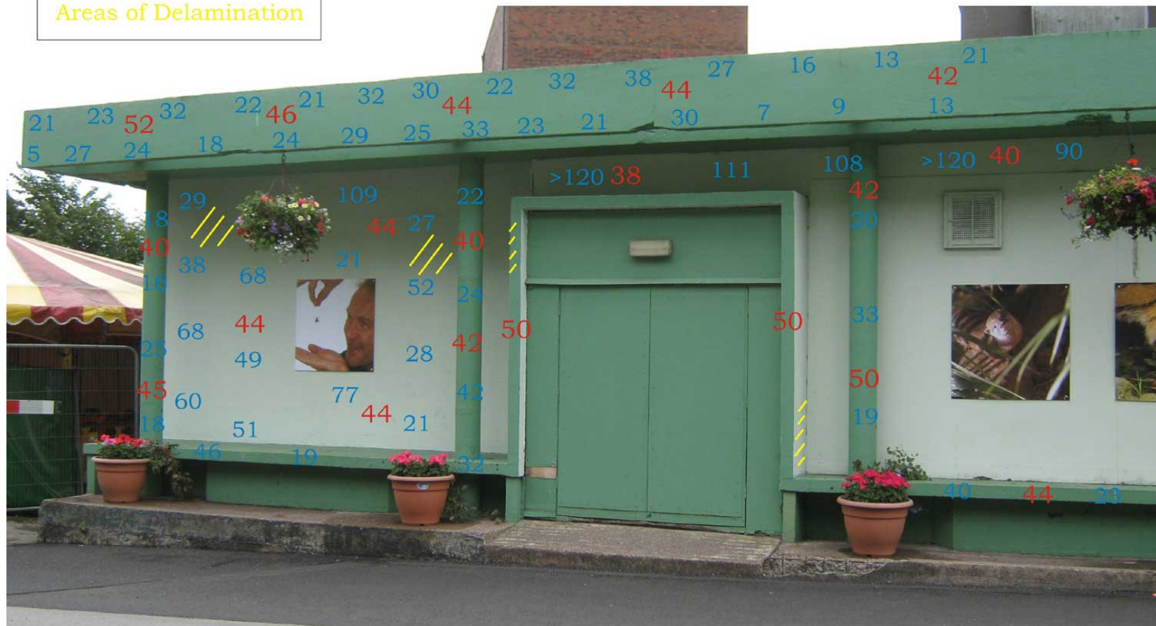
Figure A-18: Left side of the night club building (Area A)
