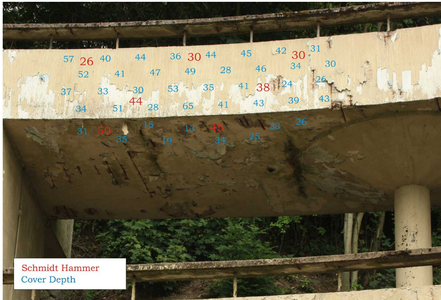
Figure A-6: Upper Platform Parapet and Soffit (Area E)
