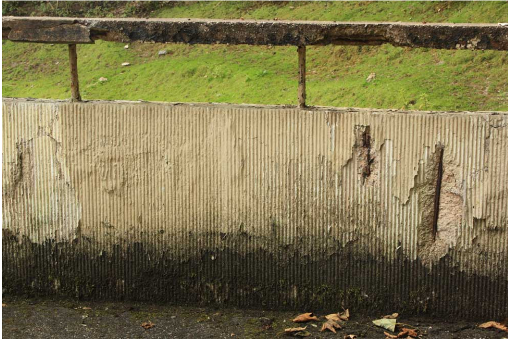
Figure 3: The corrugated finish was achieved using a thin cementitious layer applied on the base concrete.
