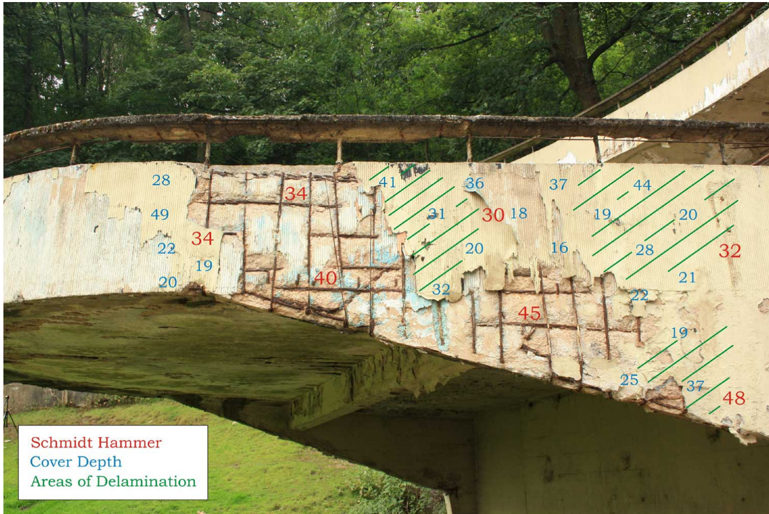
Figure A-3: Cantilevered Balcony Wall and Parapet (Area B)
