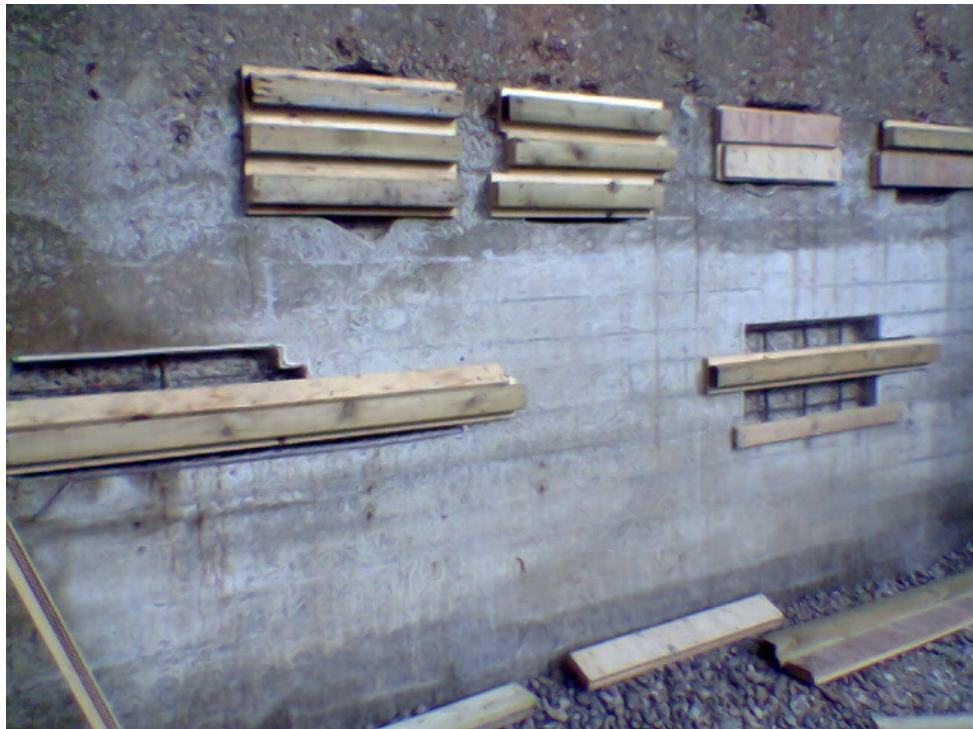
Figure C-4 Shutters fixed externally into the parent concrete to achieve board-marked finish to concrete repairs. This resulted in additional holes to be filled afterwards.
