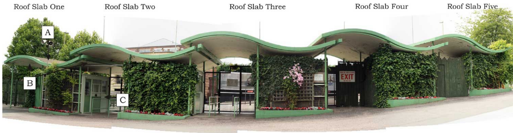
Figure A-13: Overall View of the entrance structure
