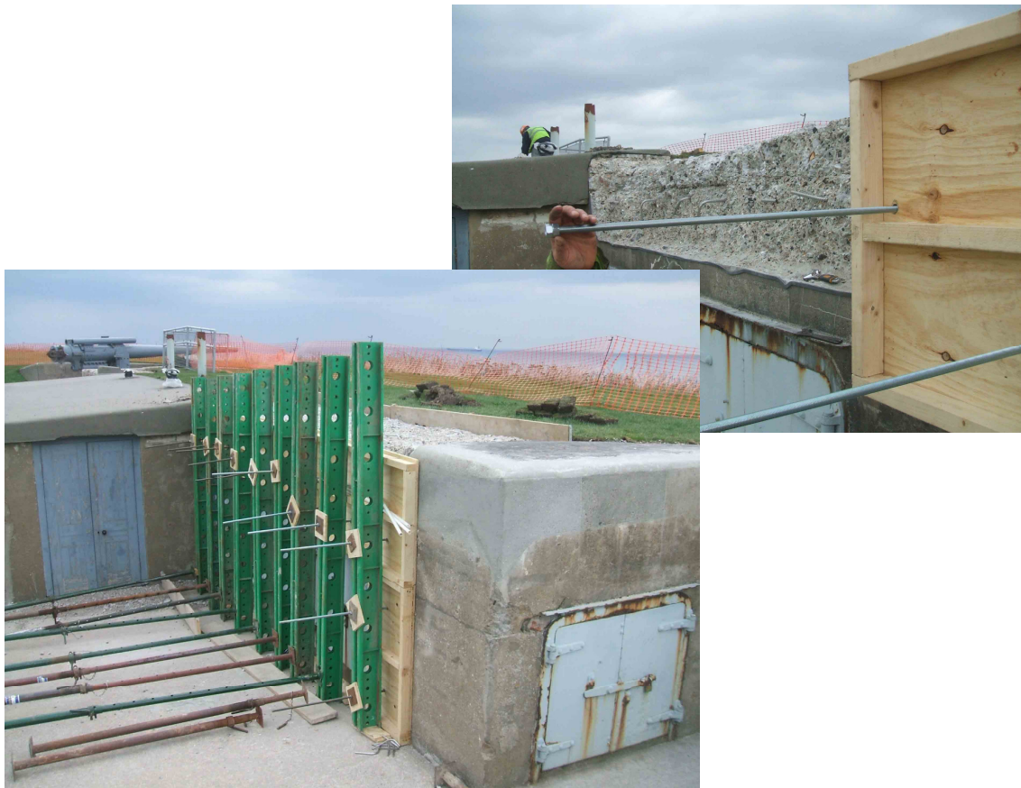
Figure C-6 Rock anchors used to fix shutters internally within the breakout.
