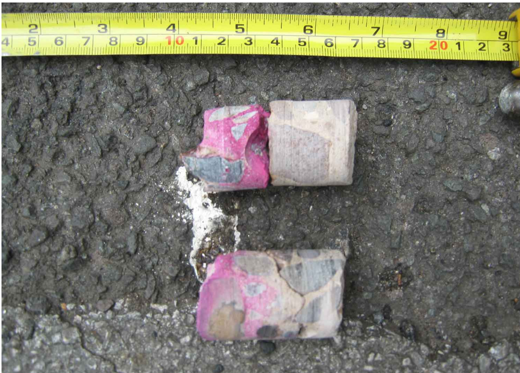
Figure A-22: Carbonation testing of two cores taken from the Kiosk.
