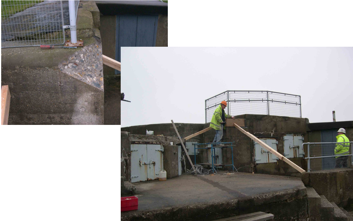
Figure C-5 Shutters fixed using external supports.
