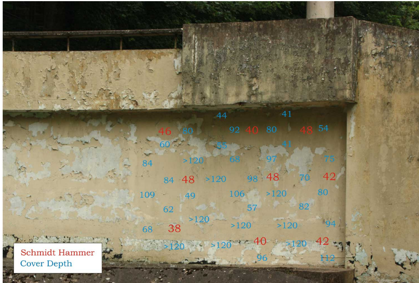
Figure A-5: Concrete Retaining Wall (Area D)
