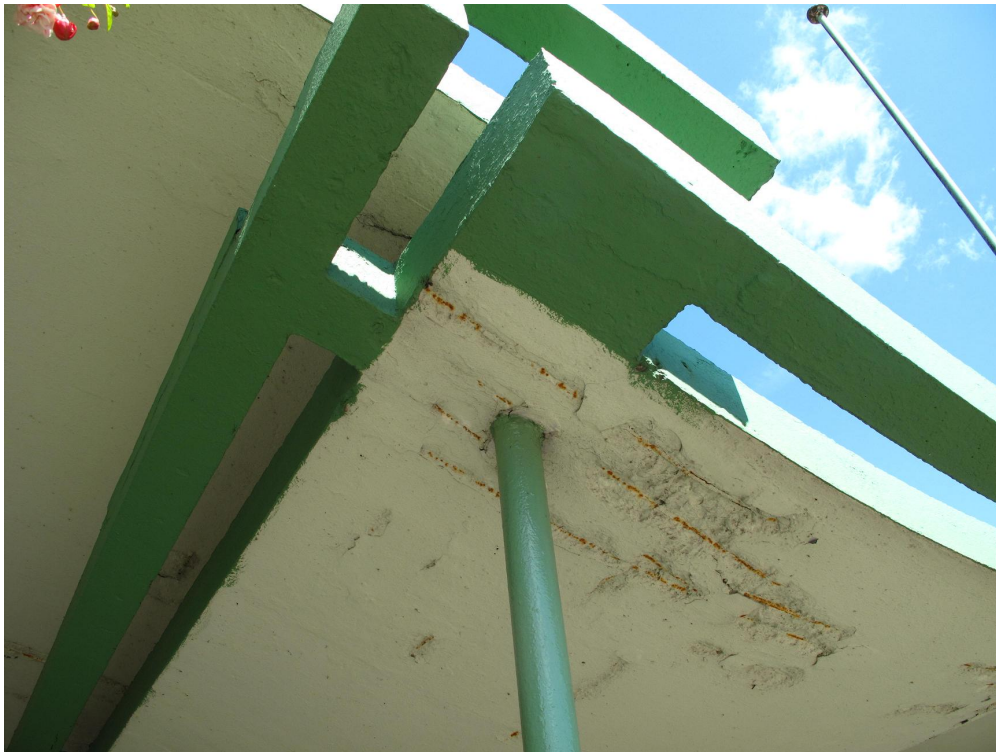
The close centres of reinforcement bars indicate a beam strip in the slab
