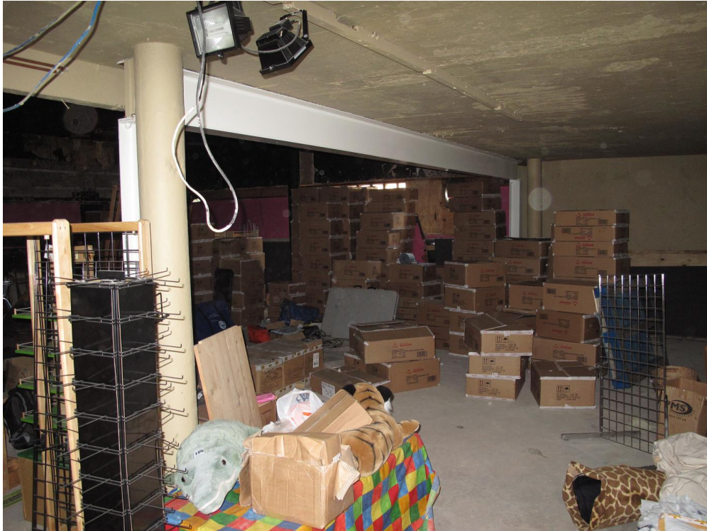
Additional steel beam and columns
