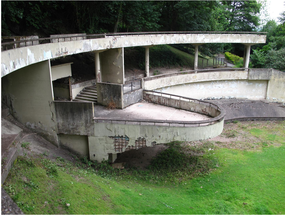
General view showing cantilevered viewing platform
