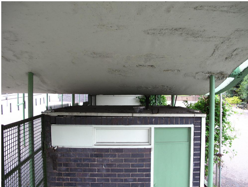
Underside of roof slab
