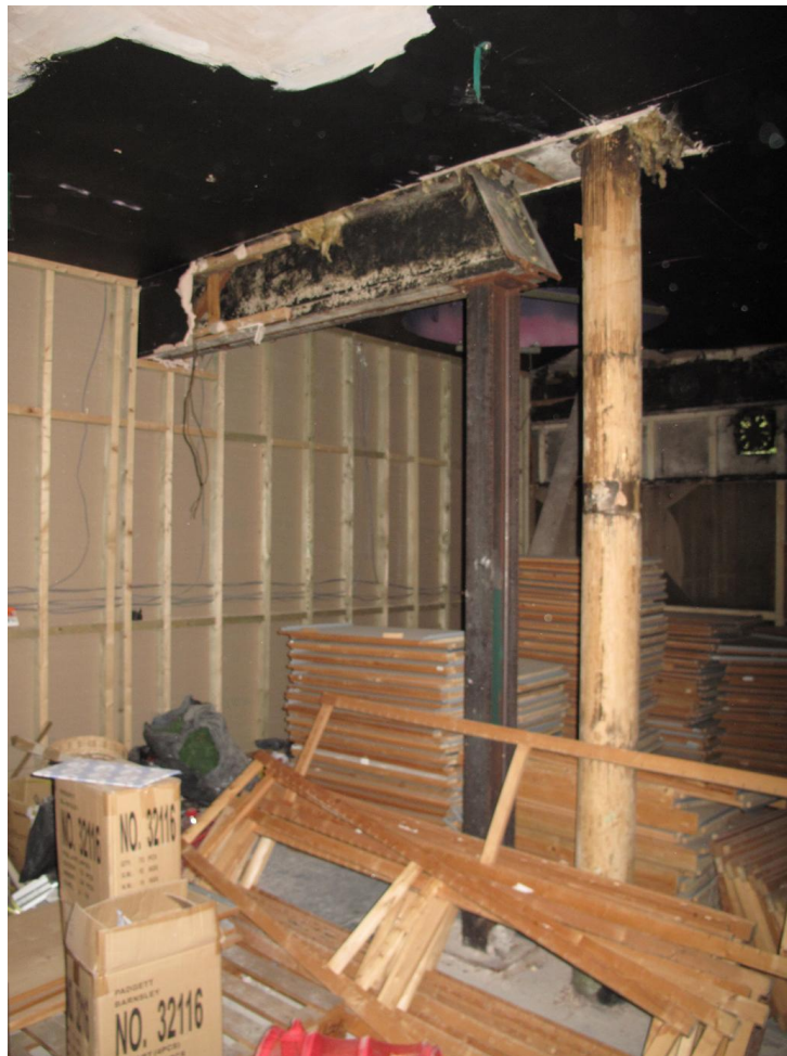
Additional steel frame where a reinforced concrete column has been removed
