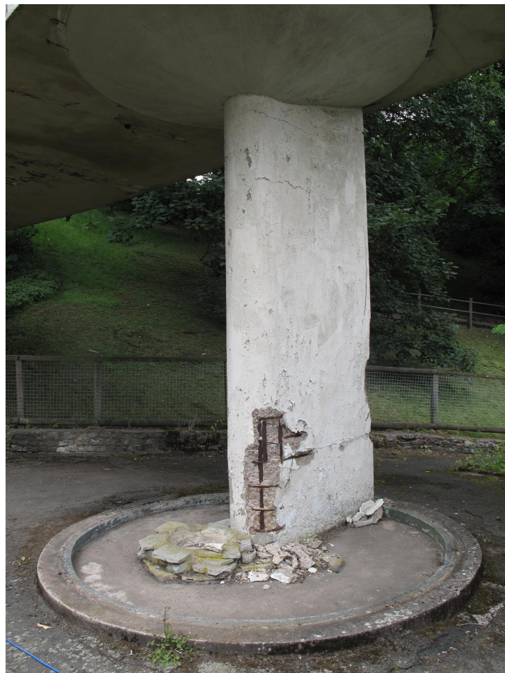
End pier provides vertical support and restraint against lateral loads & Corrosion to end pier
