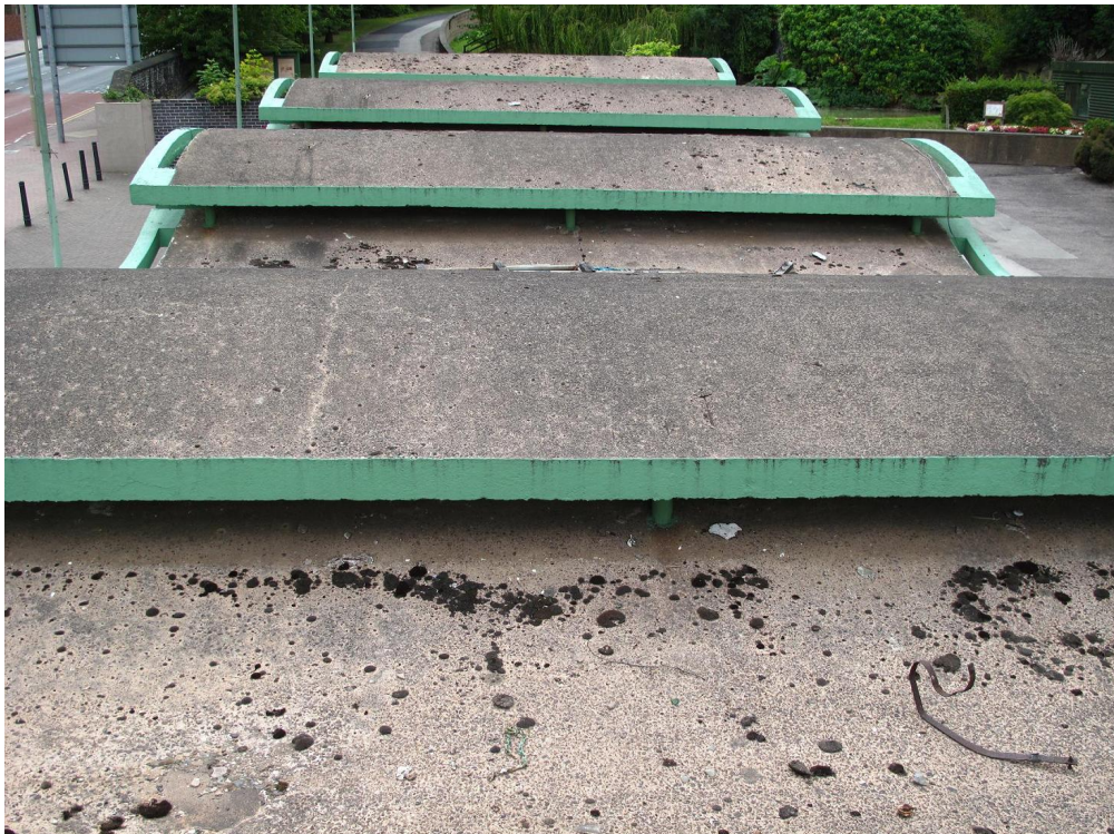
Top of roof slab
