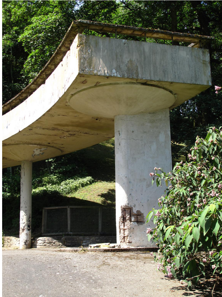
End pier provides vertical support and restraint against lateral loads & Corrosion to end pier
